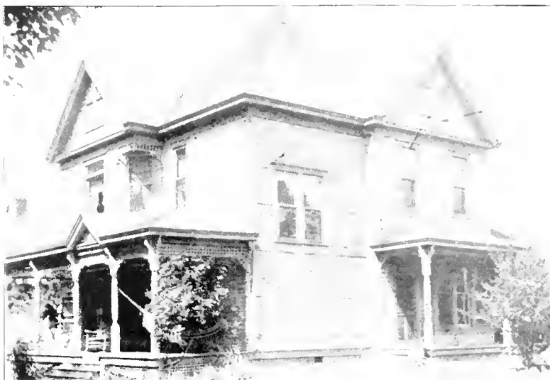
RESIDENCE OF T. N. LAKIN. North 1st Street.
